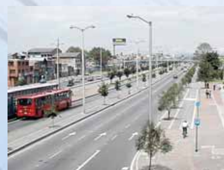
TransMilenio Bus Rapid Transit System and separation of road users in Bogotá, Colombia
