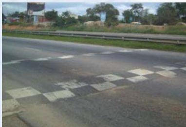
Speed hump in a built-up area to calm down traffic
